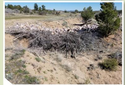
Juniper silt dam installed for erosion control. *Photo Credit: UVRWPC*
