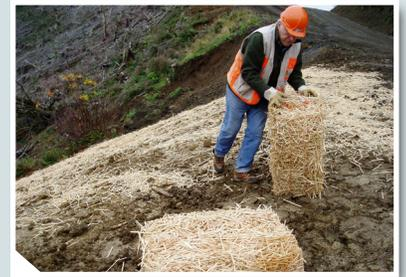
Wood straw product being hand applied for erosion control. *Photo Credit: Colorado State Forest Service*
