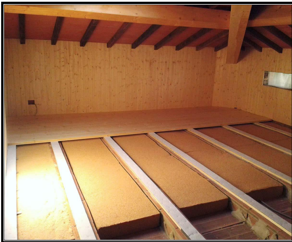
Figure 3.4 – Example of WFI Batt in Use
