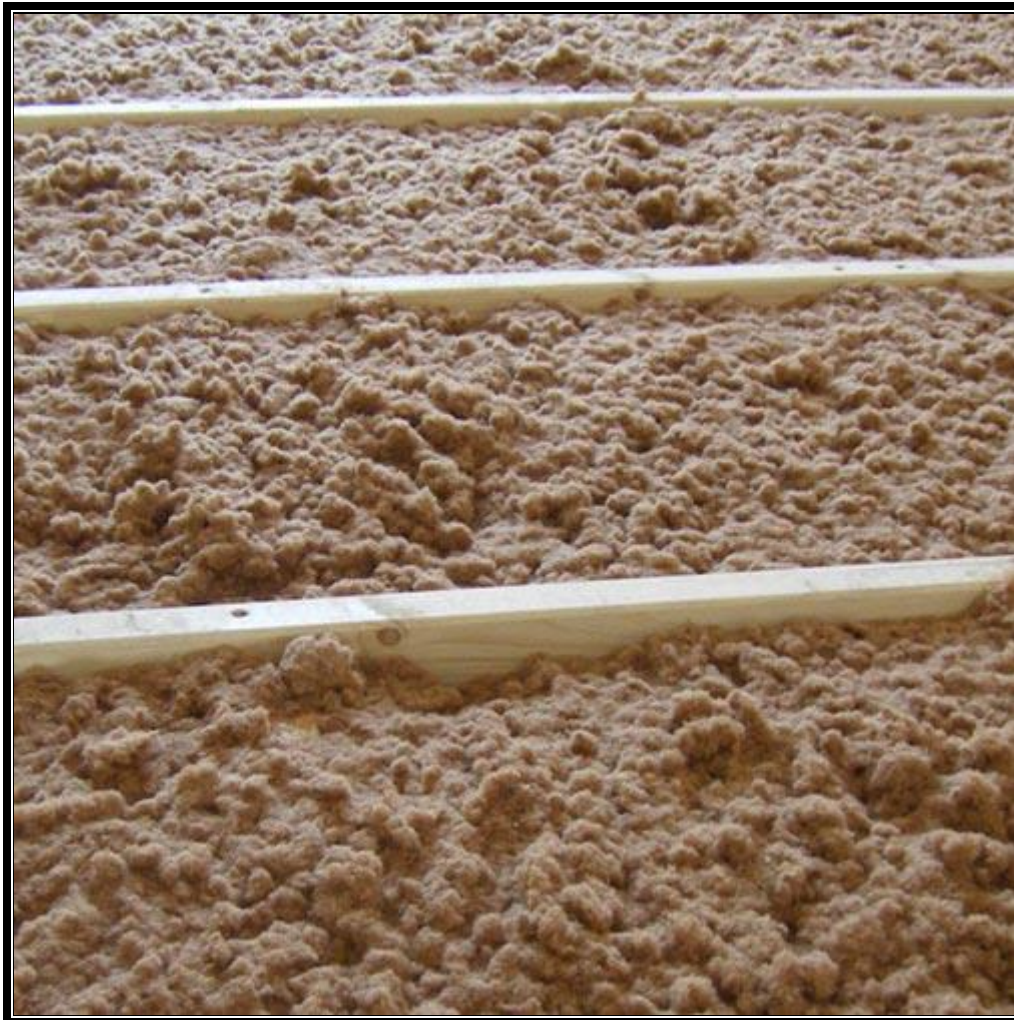
Figure 3.5 – Example of WFI Loose Fill In Use
