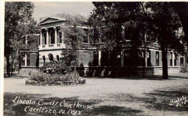
Lincoln County courthouse, c. 1940. Photo Credit: www.courthousehistory.com
