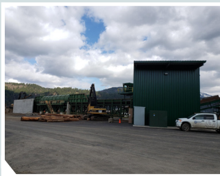
Buell's new chipping facility with infeed decks and debarker on the left and output conveyor on the right. Photo Credit: Archie Gray
