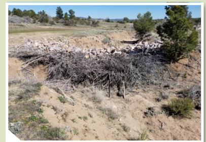
Juniper silt dam installed for erosion control. Photo Credit: UVRWPC
